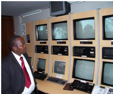
The UN facility used an old analog CCTV system and ECSI installed an IP digital video system and worked out a transition plan that would transfer from old to new systems over two weekends. To accomplish this, ECSI designed a video distribution system that paralleled the video to both the old and new system to facilitate the transition. Once the new digital video system was installed and
